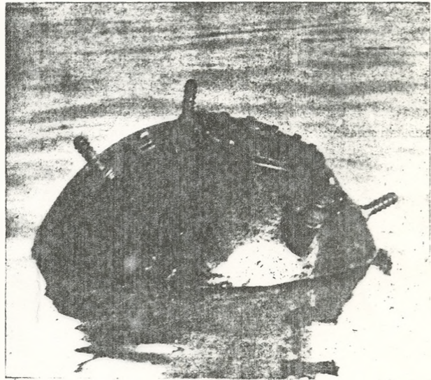
Figure 41—Mine Mk 6 Model 1, adrift
