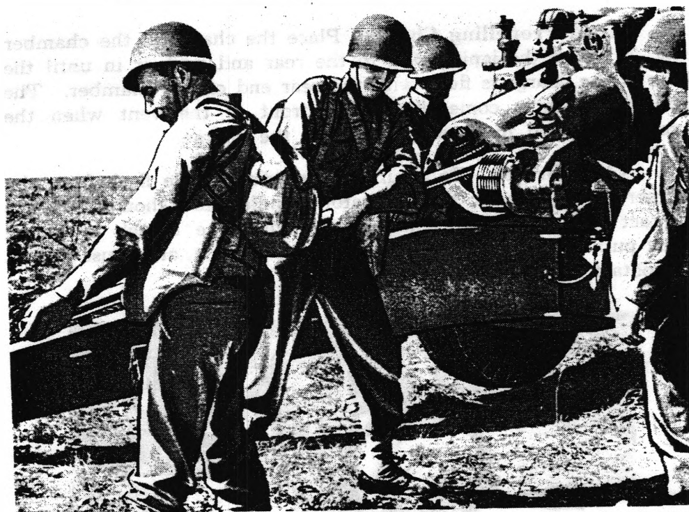
Figure 75—Ramming Projectile
