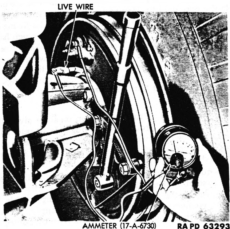
Figure 93—Checking Current at Brake With Ammeter
